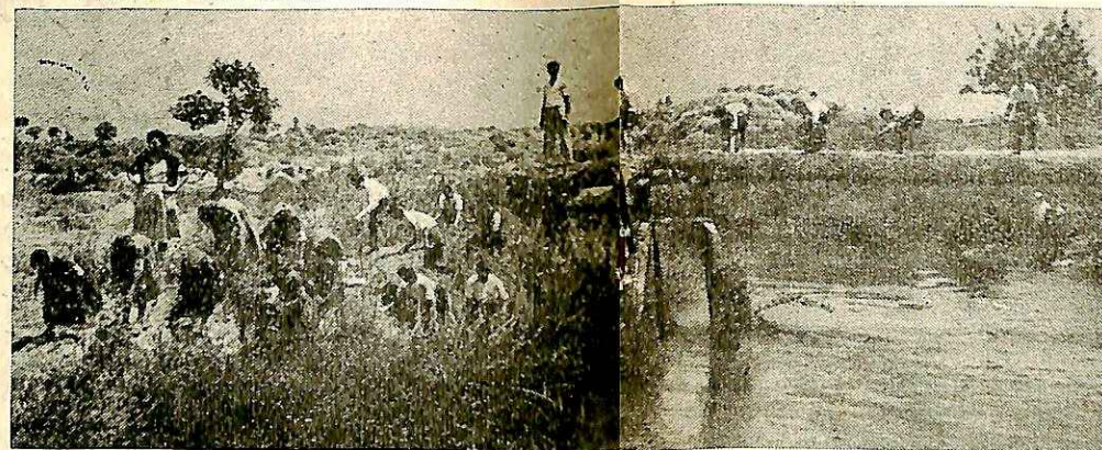
Ε.Σ.Ν. Δημ. Σχολ. Θεμέλου Πρεβέζης ἐπιχωματόνουν τὴν γέφυραν τοῦ ποταμοῦ. Juniors of Elem. School Themelon-Preveza helping in the repairing of the river bridge. ↓
