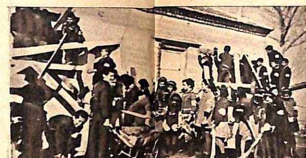
Ε.Ε.Ν. Δημ. Σχολ. Καλῶν Νερῶν Σερρῶν. Βοηθοῦν εἰς τὴν ἀνοικοδόμησιν. Juniors of Elem. School Kala Nera Macedonia helping with the Reconstruction.
