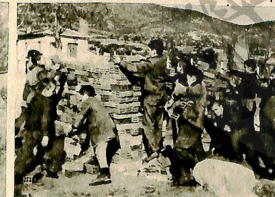
Ε.Σ.Ν. δημ. Σχολ. Βρασνῶν Λαγκαδᾶ βοηθοῦν εἰς τὴν κατασκευὴν τῶν σχολ. ἀφoδευτηρίων. Juniors of Elem. School Vrasna helping in the reconstruction of their school.
