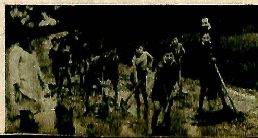
Ε.Σ.Ν. Δημ. Σχολ. Ριόλου Πατρῶν ἐπισκευάζουν τὸν δρόμον τοῦ χωρίου. Juniors of Elem. school Riolon, Patras repairing the village road.
