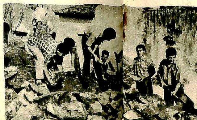
Ε.Σ.Ν. Γυμ. 'Υδρας καταστράγγιζον ἐτοιμόρροπον τοῖχον πλησίον τοῦ Γυμ. Juniors of the high school Ydra demolishing a ready to fall wall near the school.
